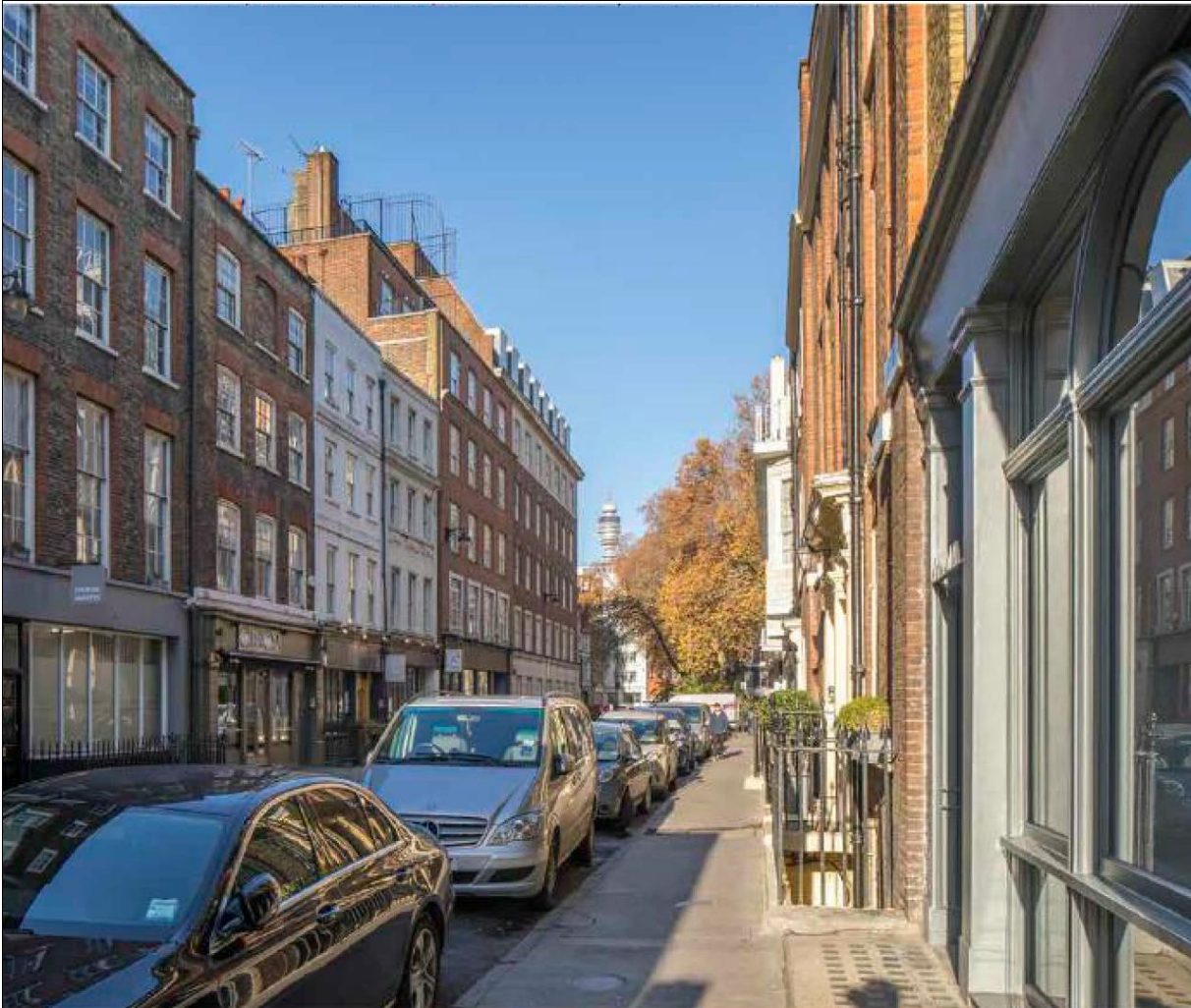
65-66 Frith Street and 31-32 Soho Square looking north on Frith Street.
